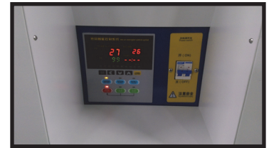
Industrial heater to generate a curing temperature inside of the machine
