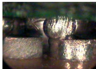
BGA – piggy back: bad alignment
